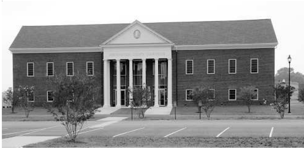
New Northampton County Court Complex
